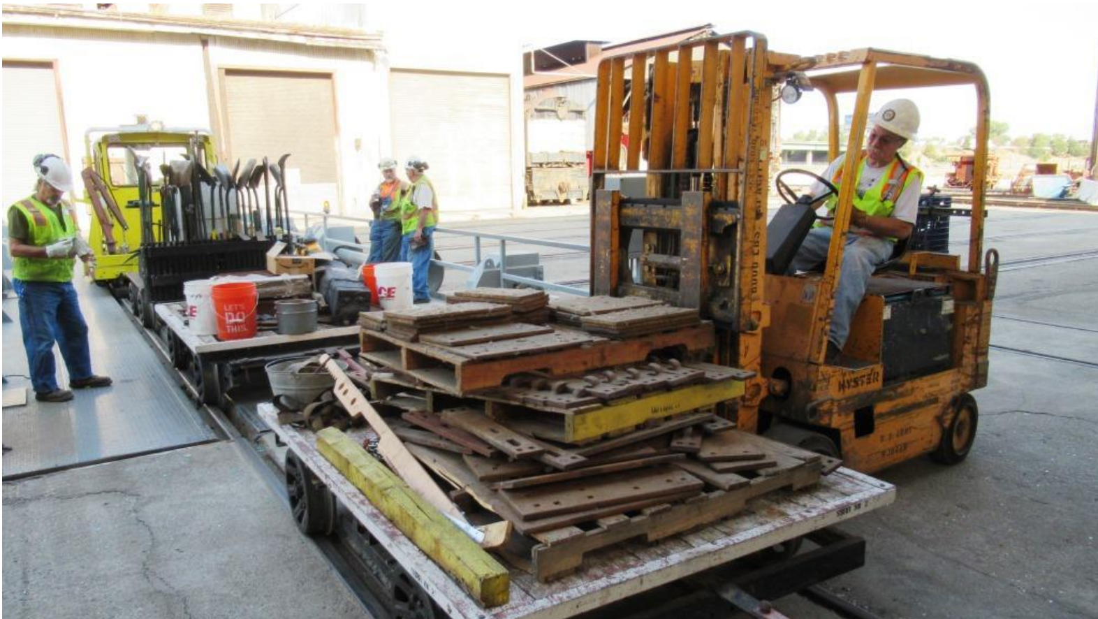
Mike H. adds another pallet of switch-plates to the flatcar
