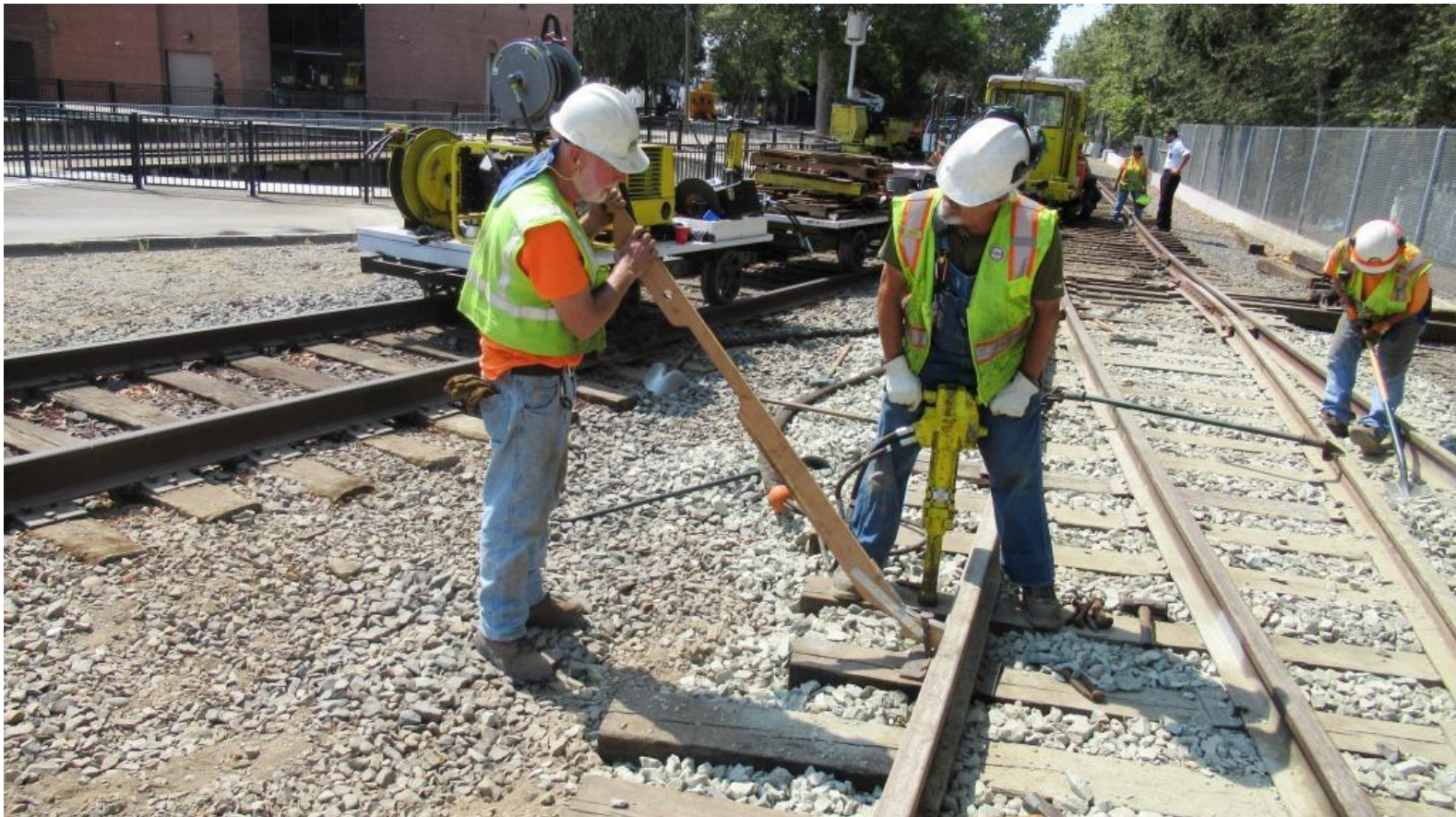
Mike M. uses the "Steve tool" to hold a spike as Ed gets ready to drive it with the hydraulic spike driver
