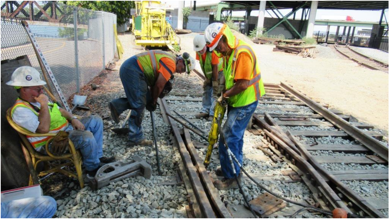
With the plates in place, Mike F. puts his back into nipping up the tie under the guard-rail as John drives spikes with the hydraulic spike driver
