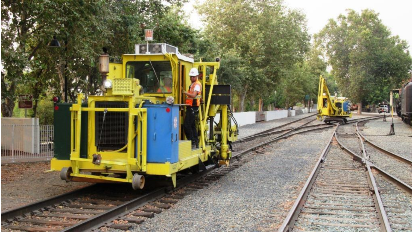
Kyle and Mike H. switch the tamper and tie-crane around
