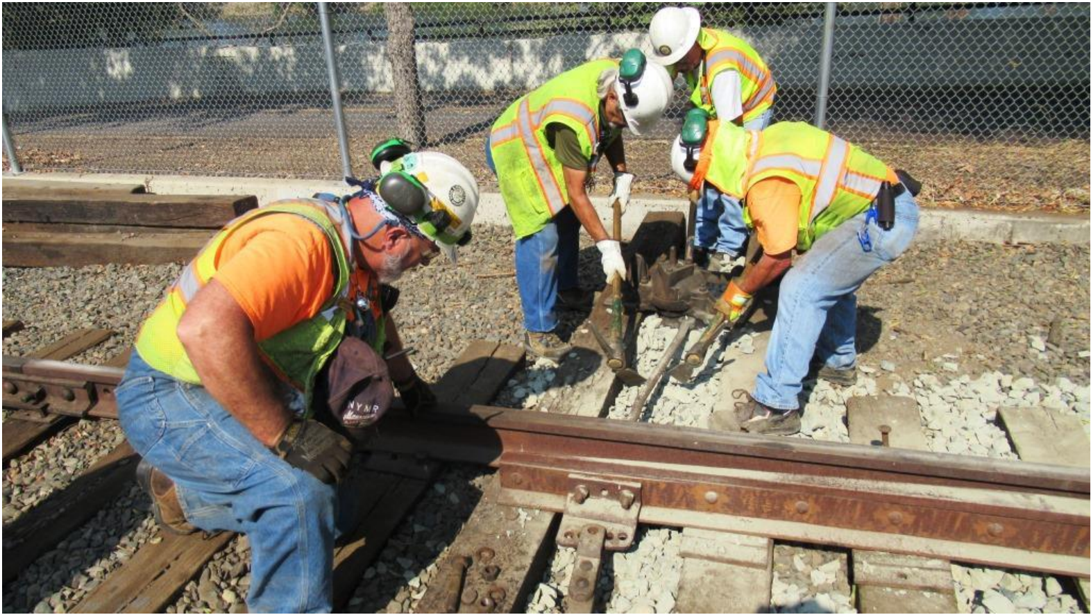
Mike F., Ed, Mike H., and Joe clear rock from under the switch-rod
