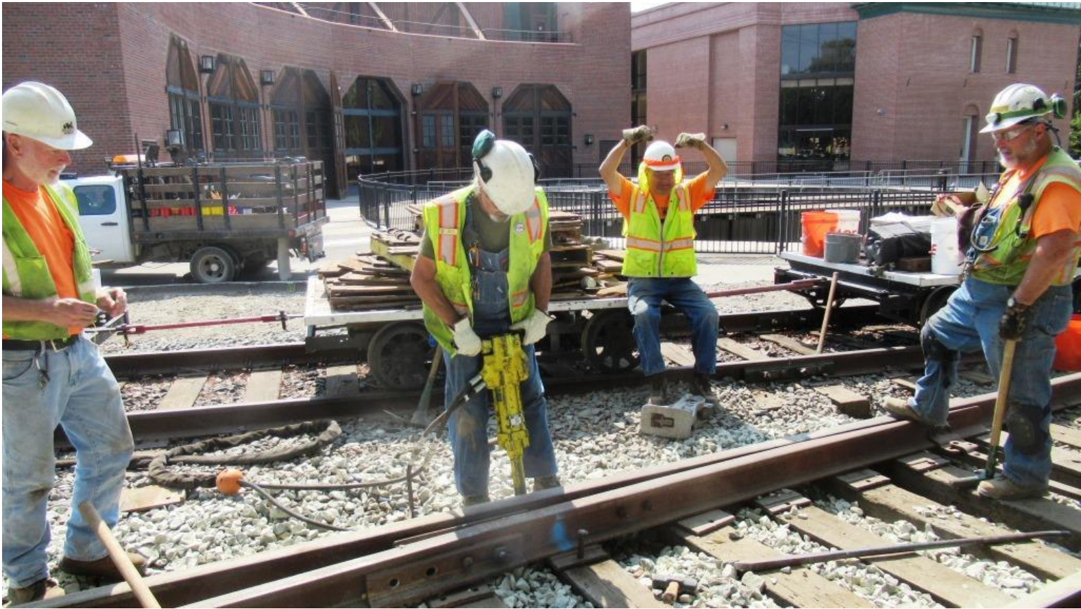
Batman keeps a close eye on Ed as he uses the hydraulic spike-driver to drive spikes
