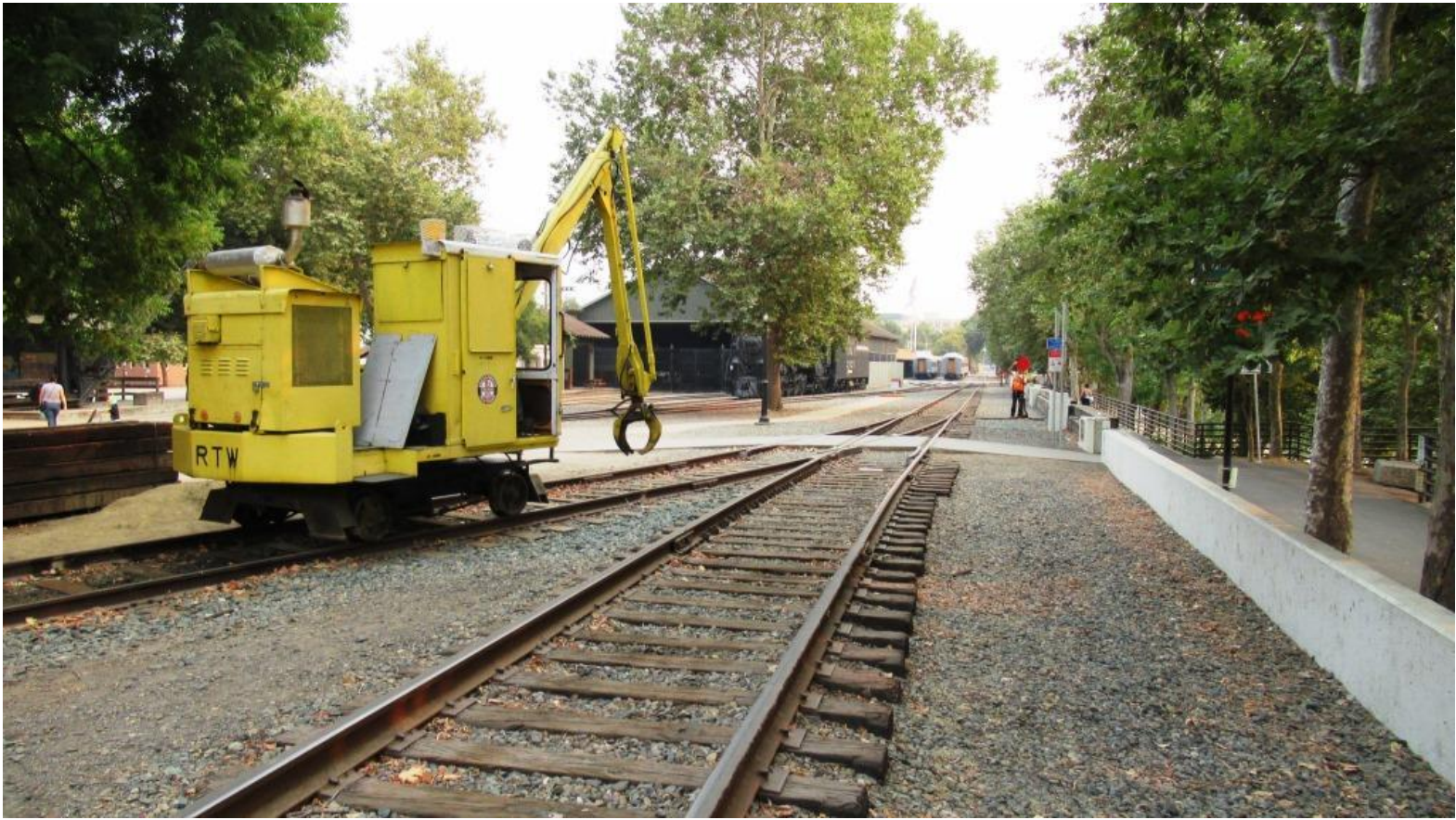
Kyle throws Switch 4 so that Alan can move the tie-crane off the North Turntable Lead
