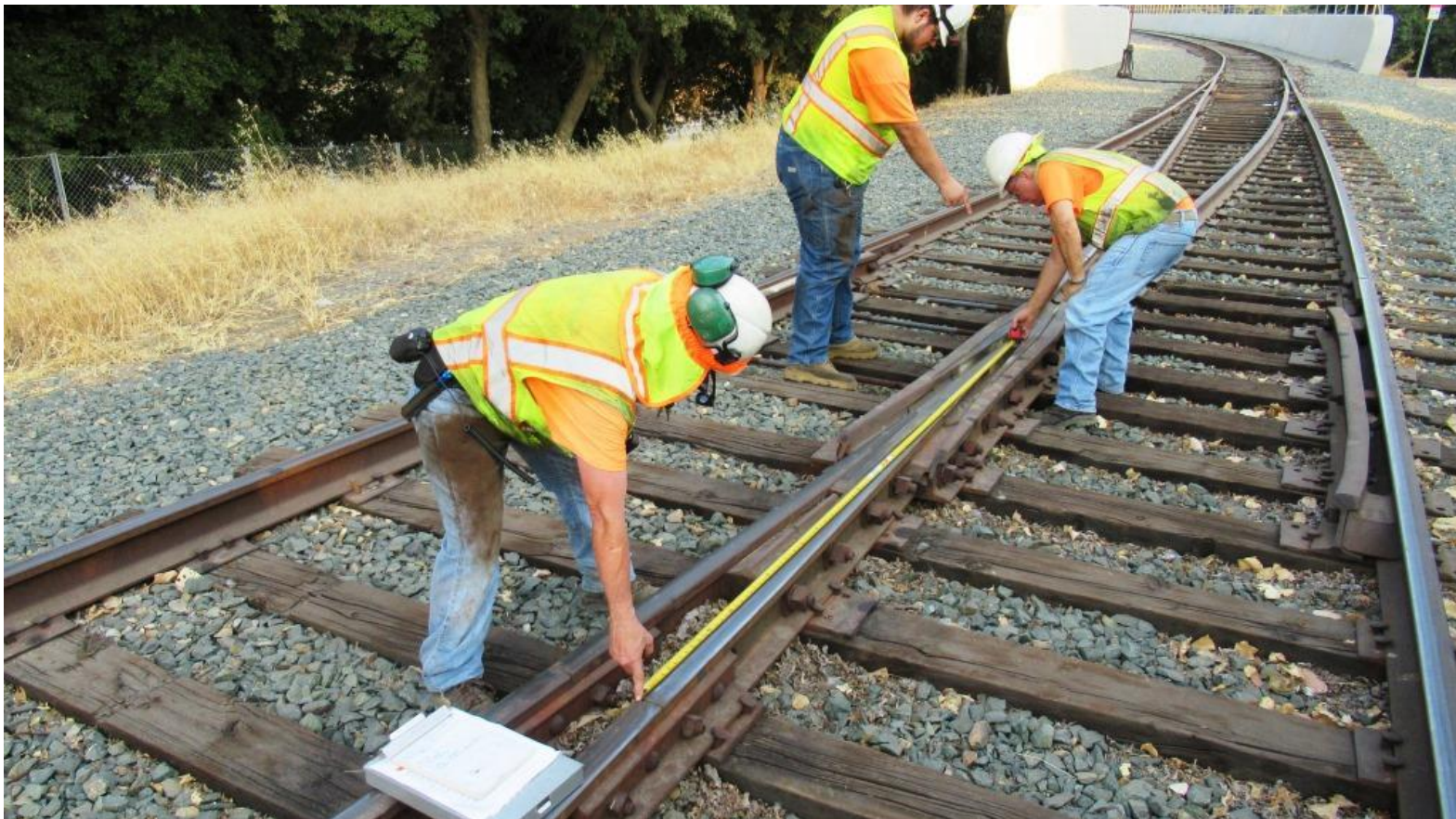
Joe, Chris, and Mike H. take measurements of the frog at Switch 20, which is identical to that being restored at Switch 19
