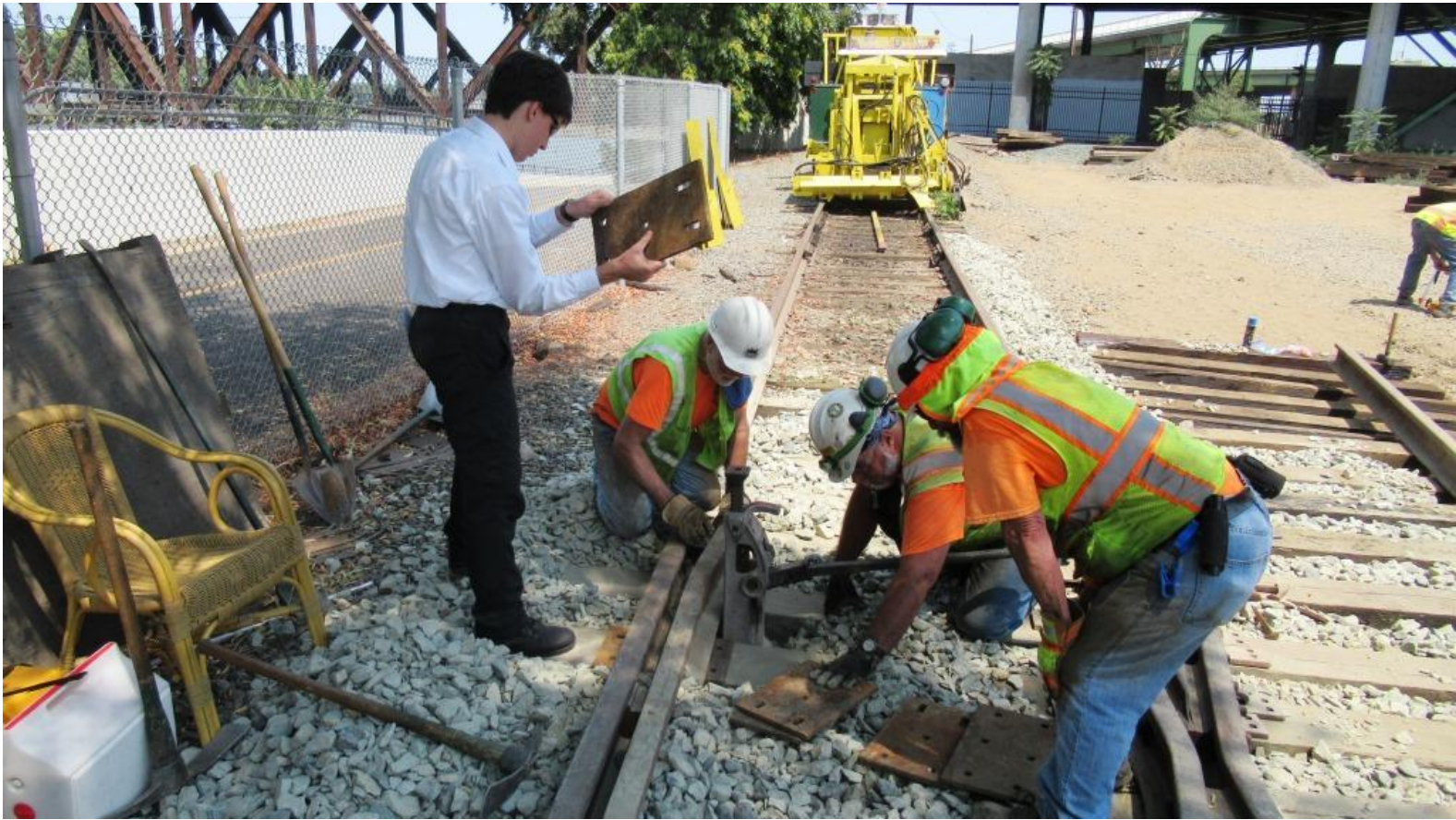
Jack, Mike M., Mike F., and Joe begin plating the guard-rail. Despite appearances, Jack is not about to “bonk-bonk” Mike M. on the head
