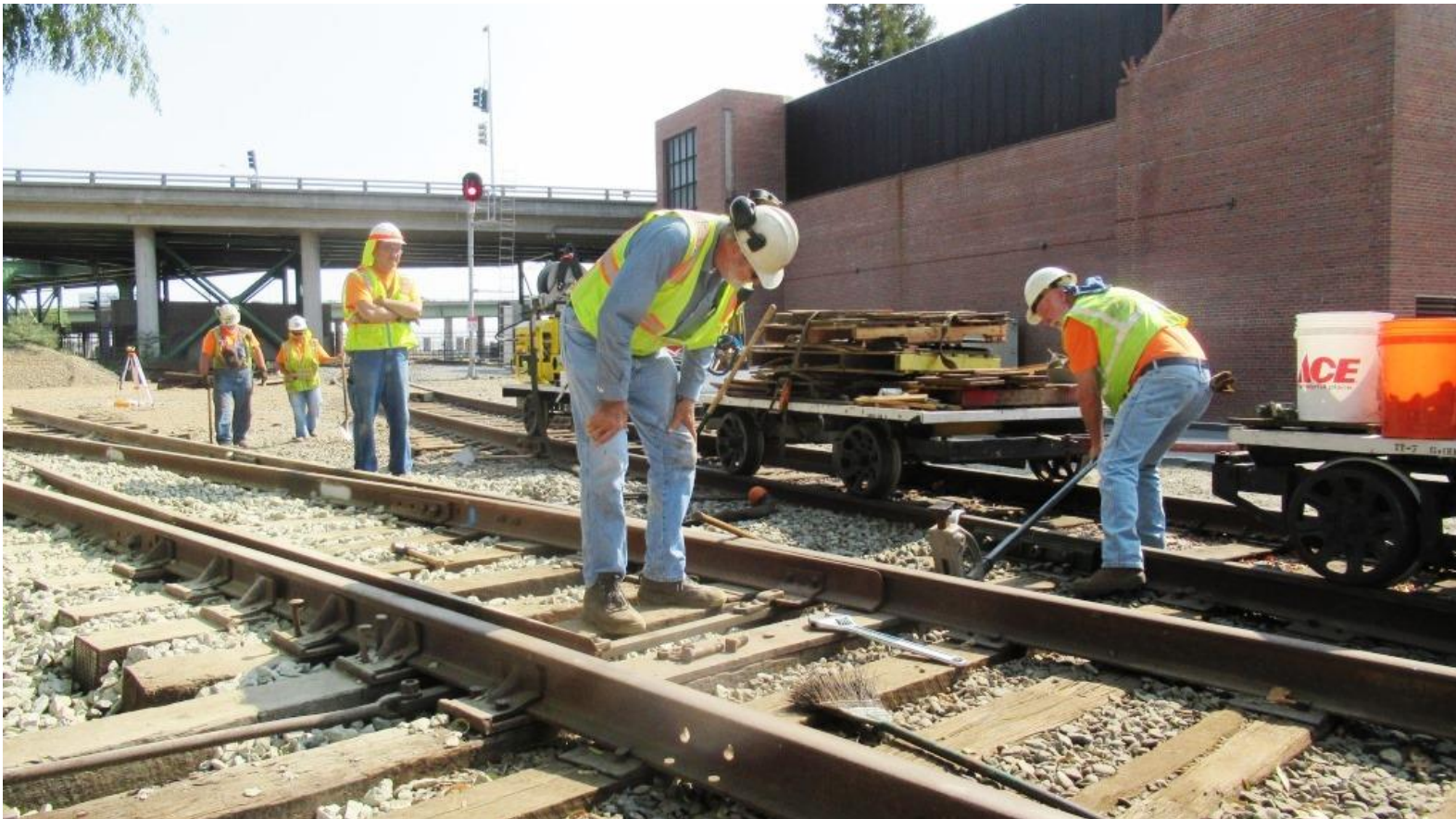
Mike M. uses a track-jack to lift the east side of the head-block as Alan checks for level
