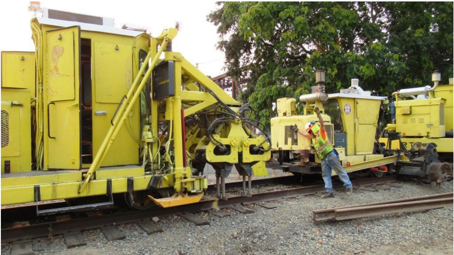
Joe guides Mike H. in the tamper to its stopping point
