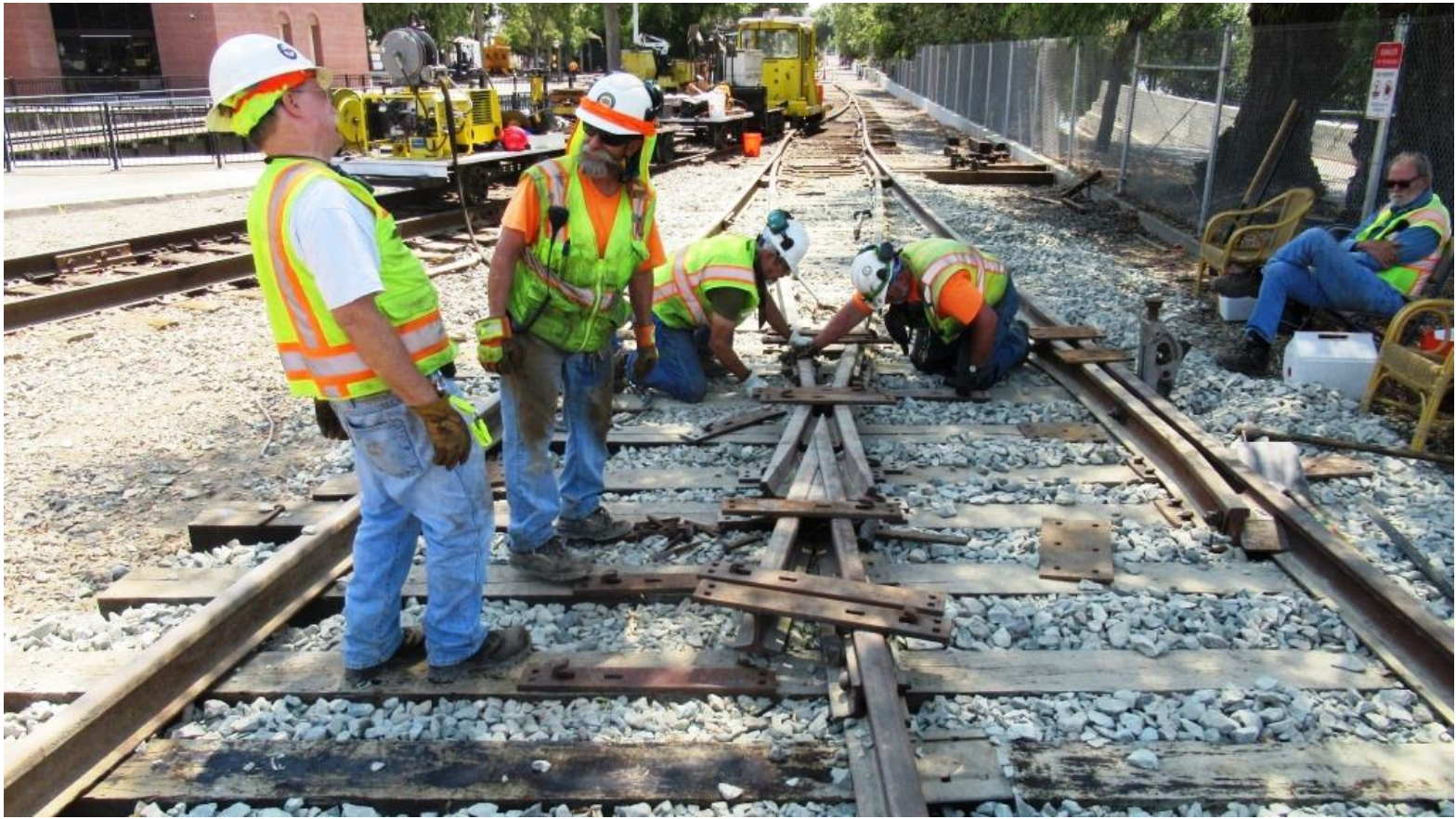
Mike H. and Joe share a funny as they work with Ed and Mike F. on figuring out the puzzle of the hook-plates for under the frog
