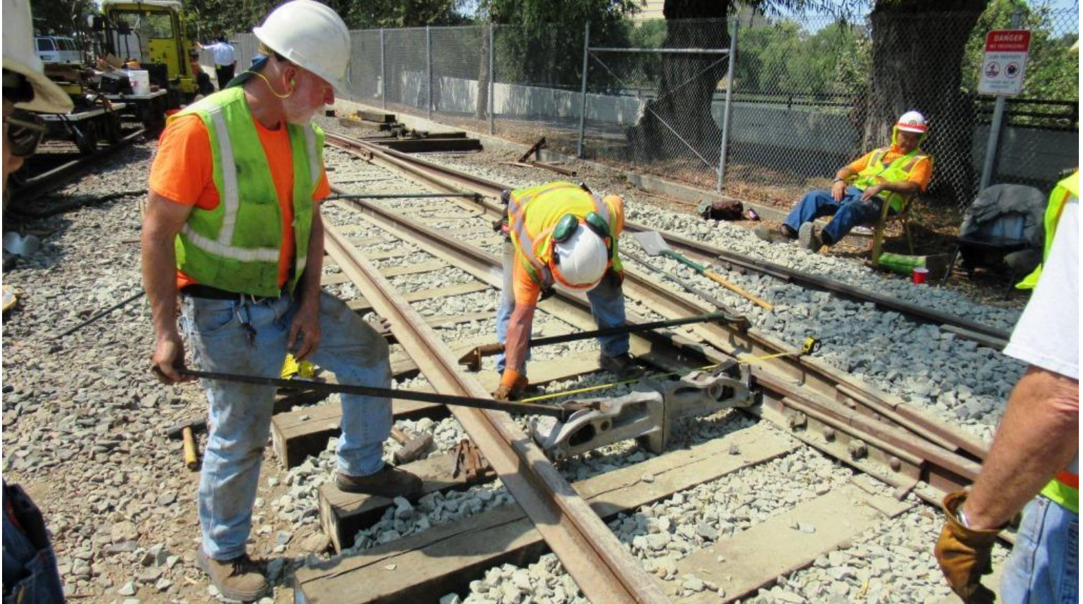
Putting a curve in rails takes effort and lots of force as demonstrated by Mike M. and Joe who use track-jacks to bow the diverging track
