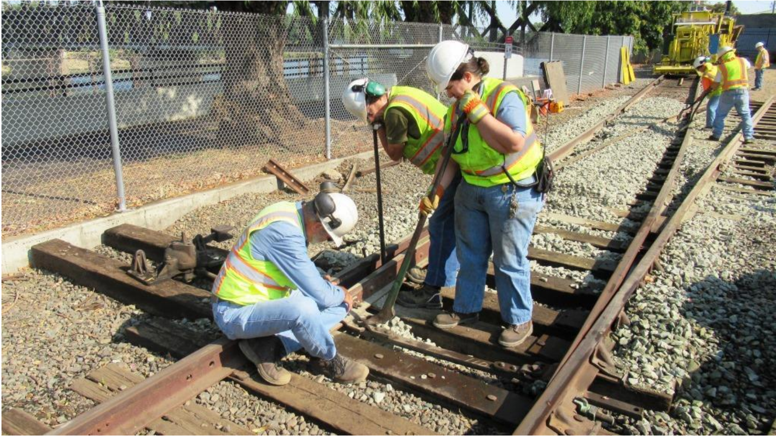
Alan, Ed, and Heather work on the positioning of the switch-points relative to the gauge-plate
