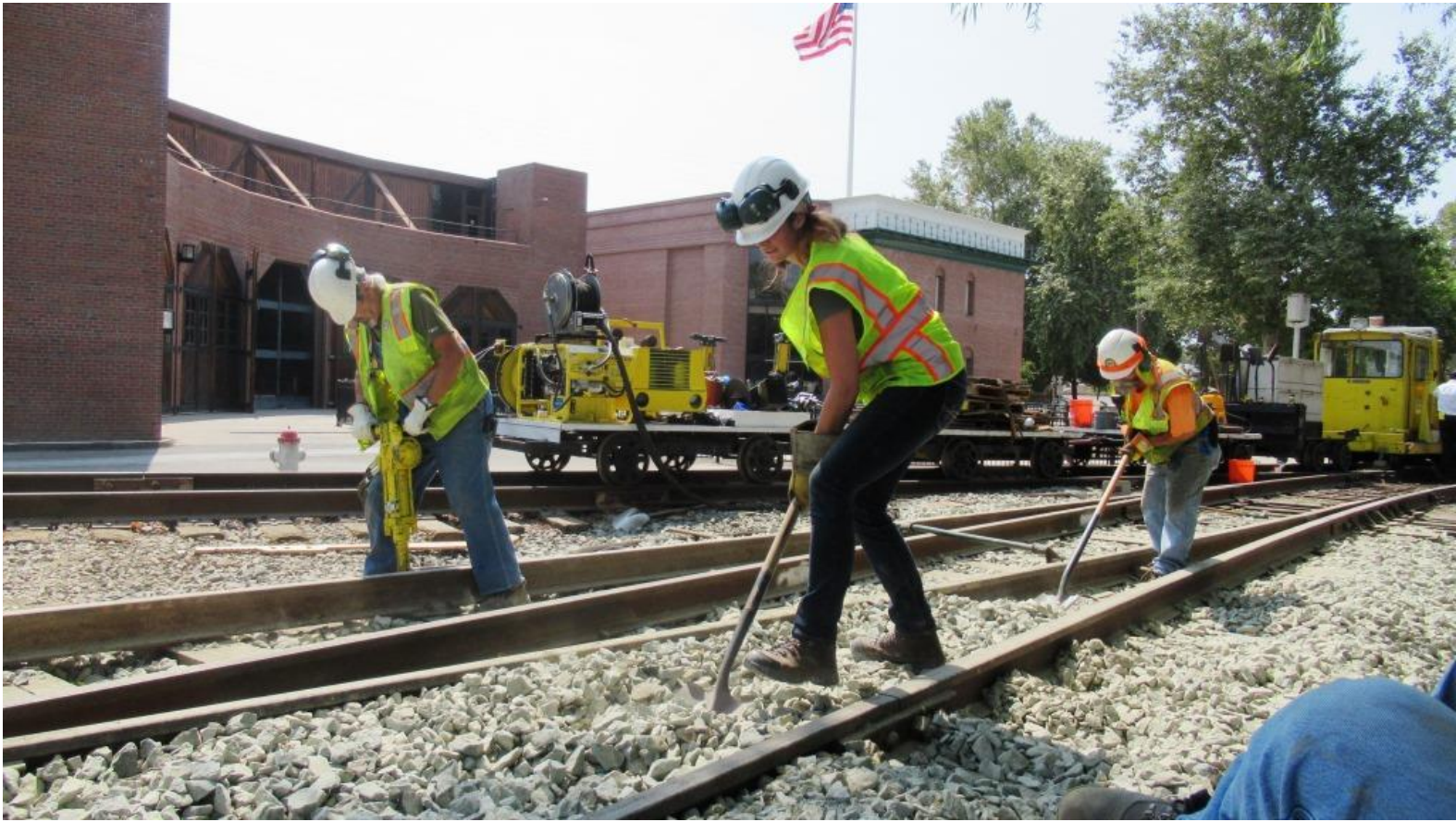
Ed drives spikes as Samantha and Joe spread rock
