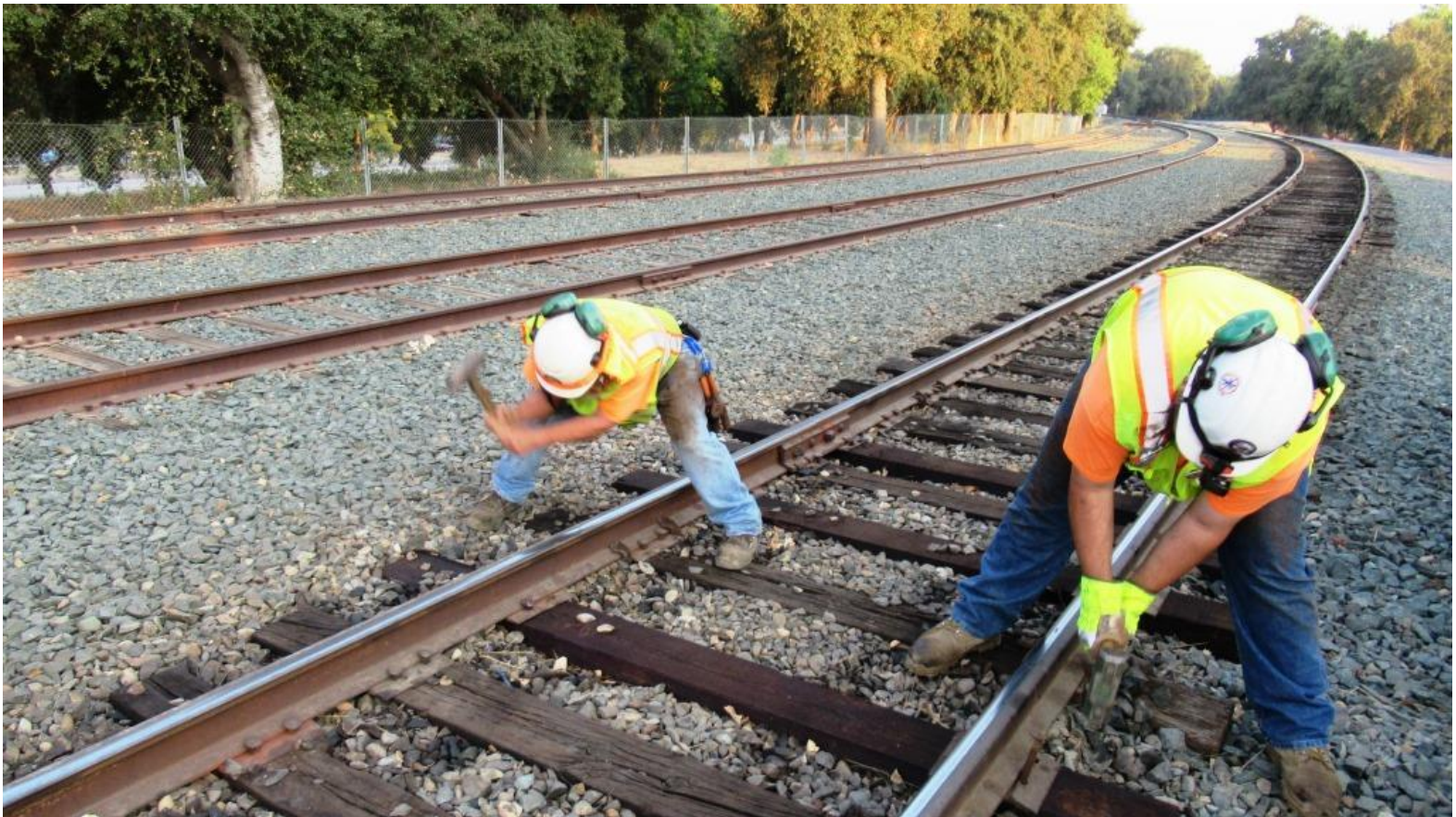
After all that fun of sorting rail-anchors, Joe and Chris try to dampen their enthusiasm by driving spikes in the 100-degree weather
